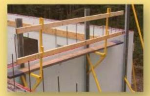
Walking platform is easily installed and the guardrail posts are removable and usable when required.
